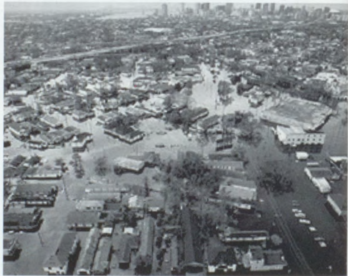
A badly flooded New Orleans, Louisiana in September, 2005, when Hurricane Katrina struck.
